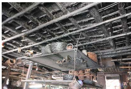
Charred ceiling seen in Mr. Kangkong Borang's humble abode as a result of the absence of outlet for the smoke from the fireplace.
